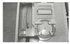
$3.6\ \mbox{Distribution}$  cable splice with pigtail and the pigtail goes the below hole of the mid-plate.
