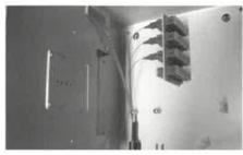
3.8 Splice the connector of pigtail to the fiber optic adaptor.
