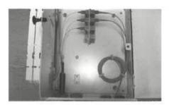
3.9 Splice the patchcord to the fiber optic adaptor.
