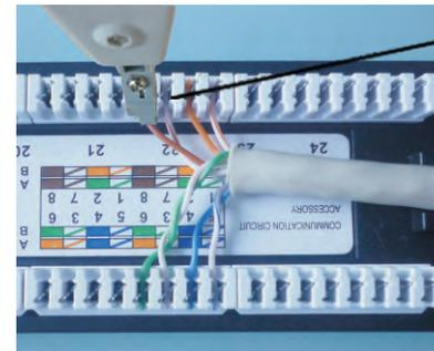
Follow the direction on the colour-coding sticker for T568A or T568B wiring. Use the impact tool to crimp and connect the wires.
