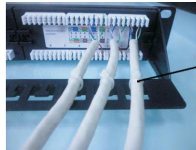
Use the Cable Tie to manage the cables, then complete the installation.
