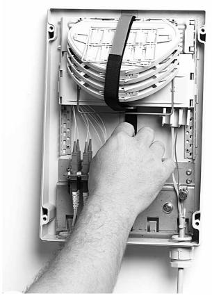
7.2 Secure the splicing trays with the Velcro strap.
