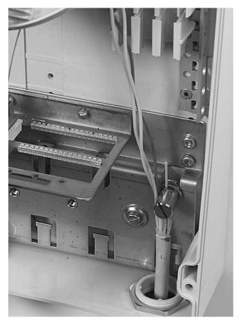
4.2.1 Pull the cable back in the correct position, the cable jacket should protrude 30 mm into the box. passing the cable strapping point.
