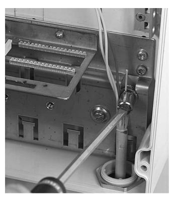
4.2.2 Insert the strength member in the strength member connector and tighten the connector with a screwdriver. If necessary remove the plastic core from the straight member till it fits in the strain relief connector.
