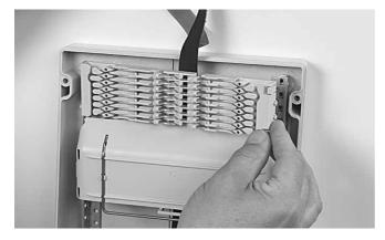
3.3.1. Take the groove plates and slide the long protrusions into the left bracket of the UMS bracket.
