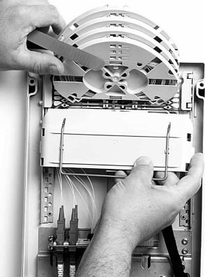
7.1 Install the FAS block cap and the retainer.
