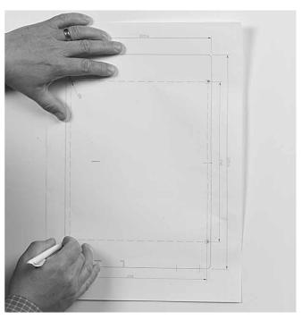
3.5.1. Place the template against the wall and mark the selected mounting positions onto the wall.
