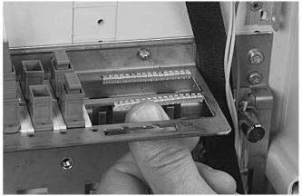
5.1.3 Install the anti movement strip (AMS) on both the slot sides of the patch panel.
