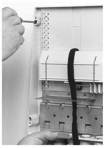
3.5.3. Hold the base part onto the wall. Insert the screws and tighten.
