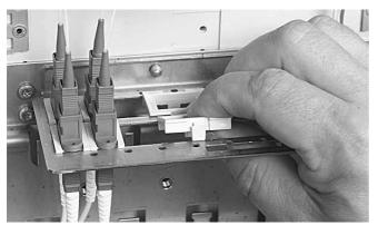
5.2.1 A Kevlar termination adapter has to be installed in the patch panel. Push the adapter from the top in the patch panel, an slide it in position. Each adapter can contain two KTUs.
