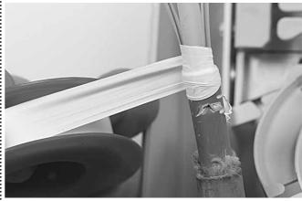
$4.1.3.2\,$  Protect the transition from the cable to the tubes with a few layers of Teflon tape.
