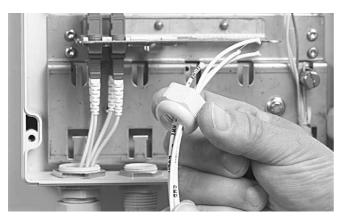
5.2.2 Slide the pigtail gland nut over the pigtails and feed the pigtails through The gland and the patch panel adapter.
