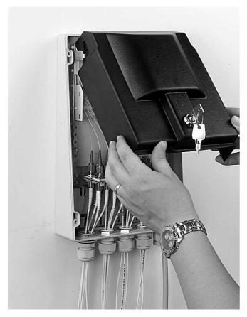
$7.3\,$   $\,$  In case of a inner cover hook the cover over the brackets and secure with the key.
