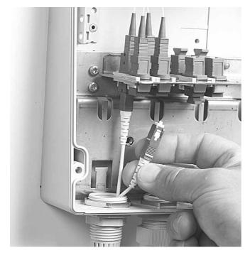
5.1.5 Remove the pigtail gland seal and nut, feed the jumper connectors through the gland and mount the connectors to the adapter on the patch panel.
