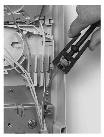
4.3.3 Cut and remove the excess of the loose tube and clean the fibers.
