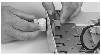
3.2.3 Install the glands in the selected ports by tighten the nut on the inside of the box, do not forget to install the rubber ring on the outside of the box.
