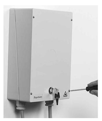
7.4 Place the cover on the box base and secure the cover with the screws.
