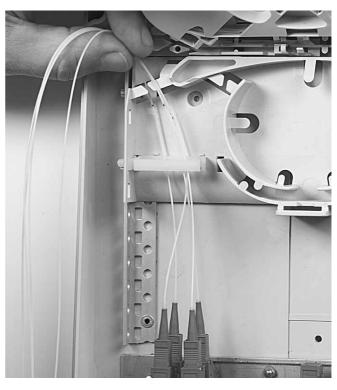
5.1.4 Mount the pigtail connectors in the adapters and route the pigtails to the splicing trays.
