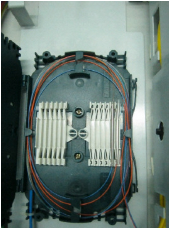
3. Splice the optical fibres
